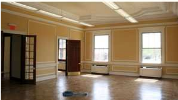
Ken Wyner Photography The restoration program involved significant reconstruction of the first-floor living room, converted to an open office area. The work included removal of the hung ceiling grid and faux-pine paneling; making structural repairs and installing HVAC pipes for the
