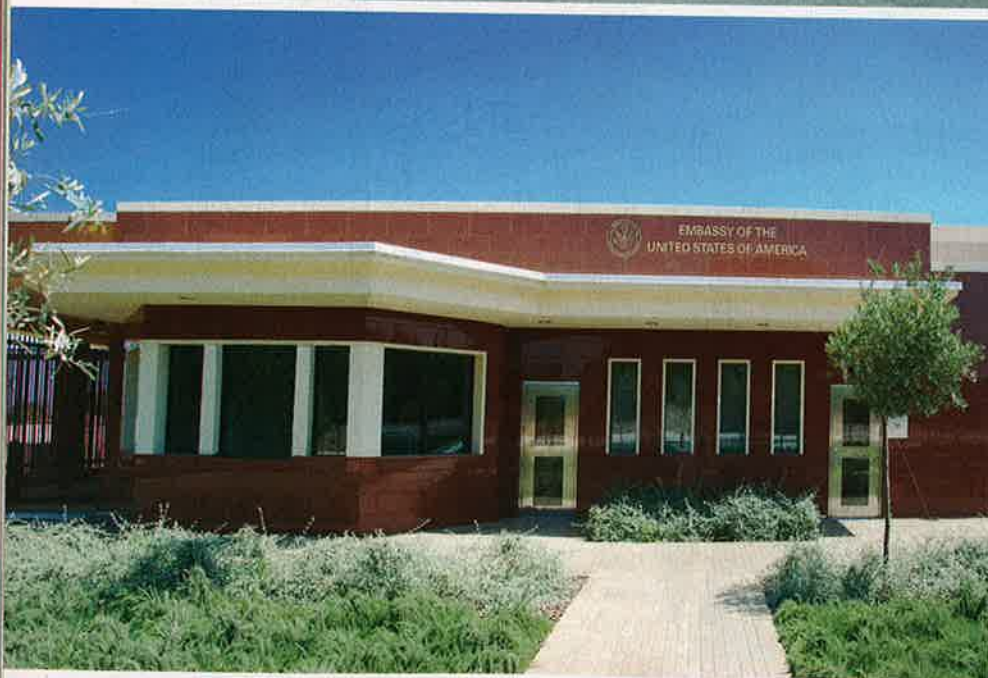
Imperial Red granite clads the exterior facade of the controlled access building.
